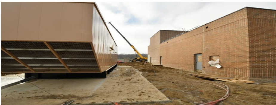
New standby generator and Headworks Building. Estimated startup date - summer 2020.
