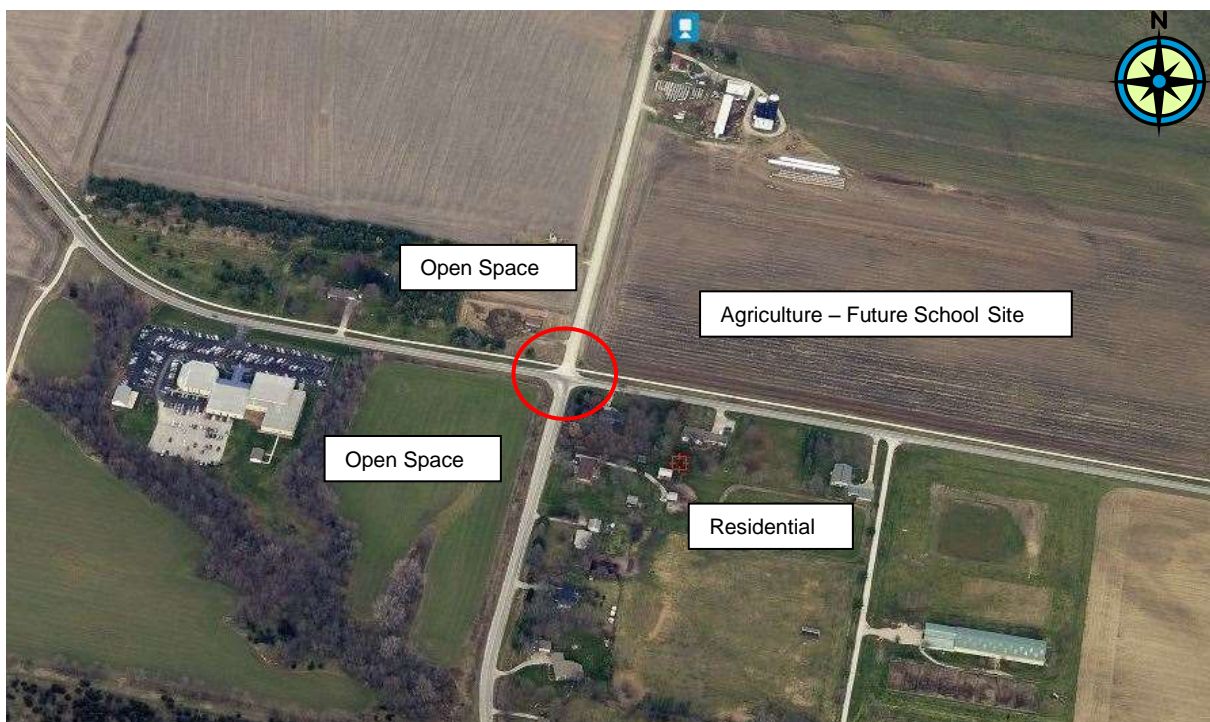
Figure 6 - Dubuque Street NE / North Liberty Road intersection
