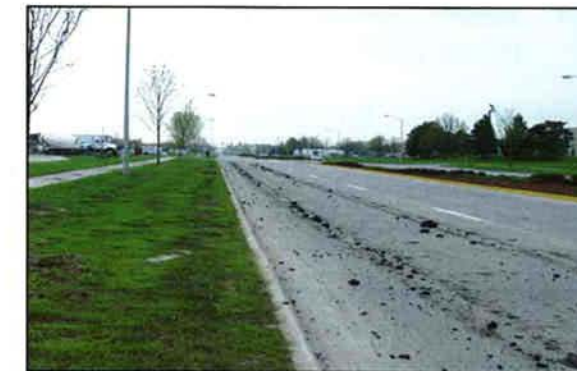
Mud tracked onto streets from construction sites will be transported to surface water via storm drains.
