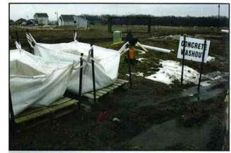
Concrete washout materials must be contained where waste concrete can solidify in place and excess water can safely evaporate.
