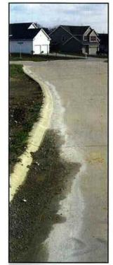
This trail of white residue is evidence of concrete washout flowing to the storm drain and into the stream.
