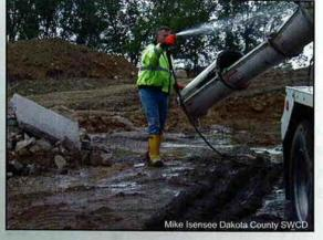
Do not wash out concrete trucks into storm drains, open ditches, streets, or streams.
