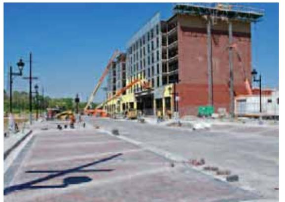
Homewood Suites by Hilton under construction along East 2nd Avenue. Permeable pavers (bricked area in foreground) allow stormwater to infiltrate to the soil below.
