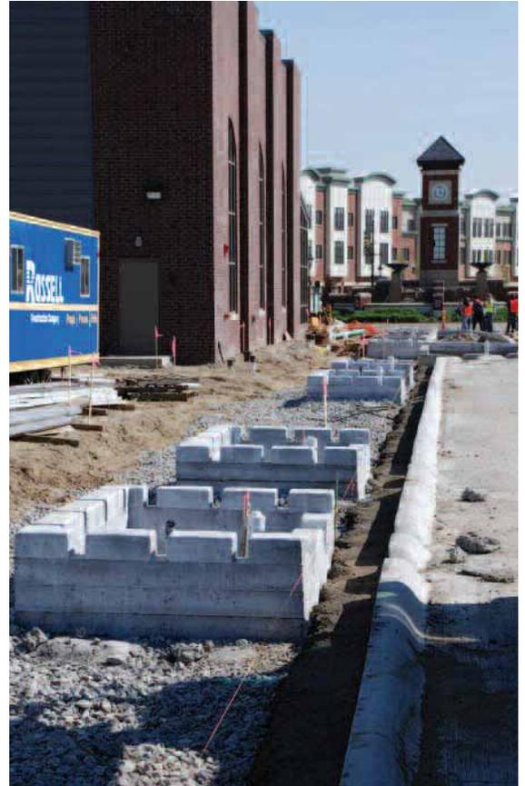
Stormwater planters, which will be landscaped and will capture and infiltrate stormwater runoff, line Quarry Road Extension next to Backpocket Brewery.
